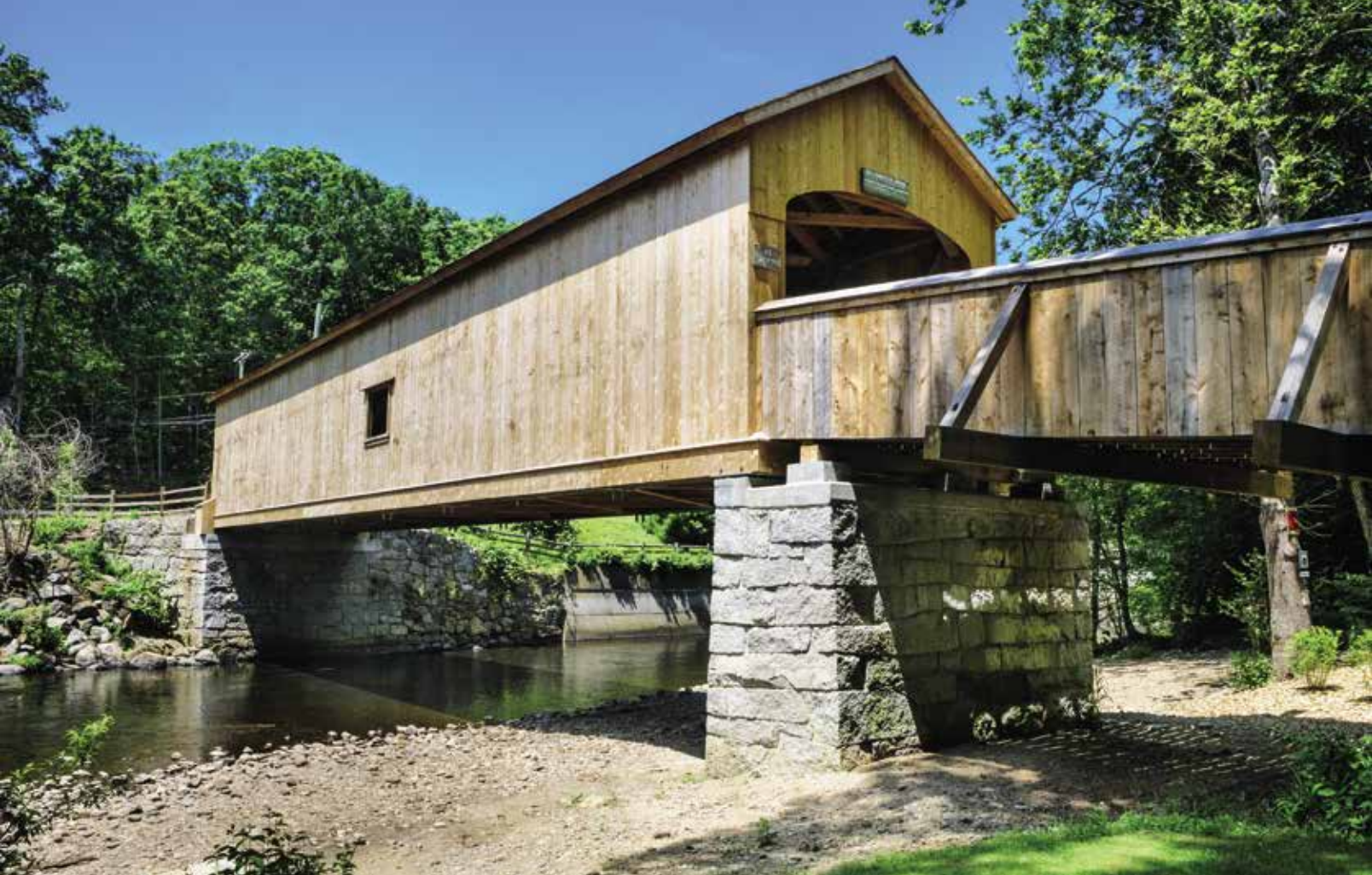
The Comstock Bridge is a single-span Howe truss design with a total length of 80 feet. It is closed to vehicular traffic but carries a foot trail over the Salmon River in the town of East Hampton, Connecticut. This historic bridge is a 2012 renovation of the original, which was built in 1791 and repaired by the Civilian Conservation Corps in 1936.
